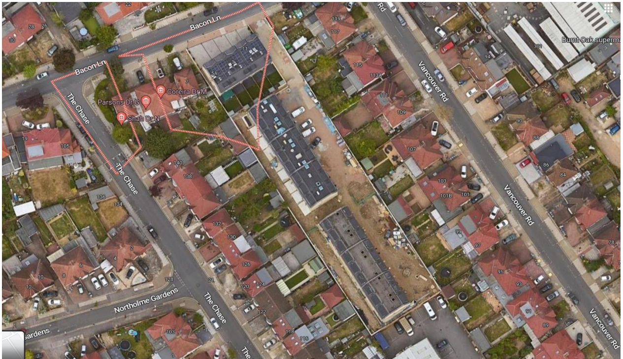
Aerial photograph showing the development with the built dormers
