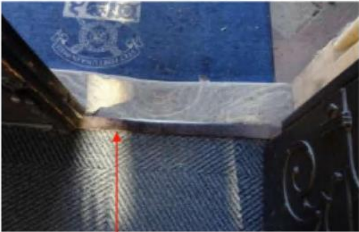
Metal threshold strip at rear of the stone step
