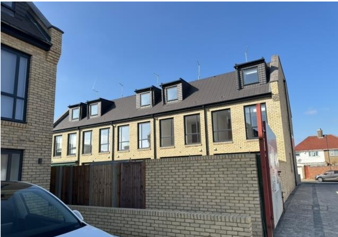
Rear of Block A – built rear dormers
