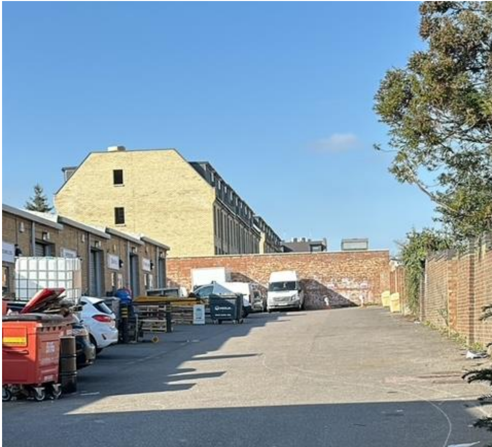
Block C – view from south looking back at development from Mill Yard Industrial Estate, Columbia Avenue
