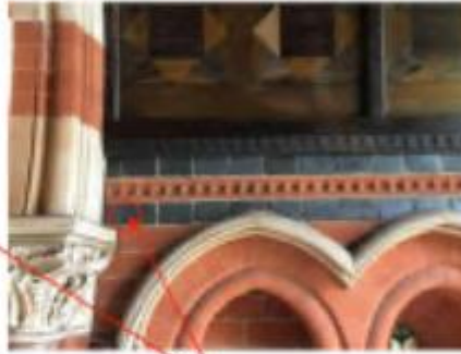
cctv camera location
